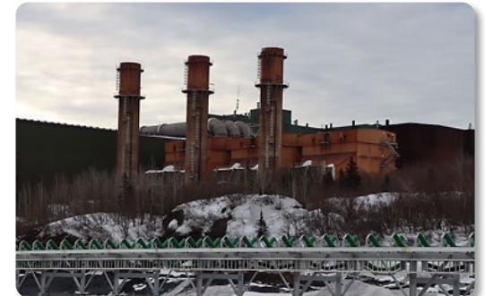
Pointe Noire Pelletizing Facility
