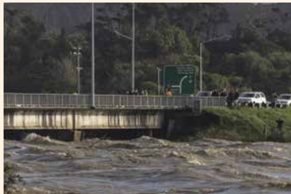
Buller River Bridge – Westport (Source: C McLachlan)
