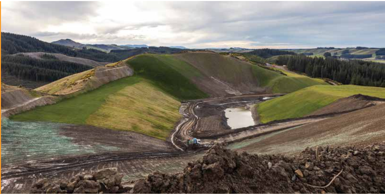
Engineered landform (ELF) in progress at Canterbury mine
