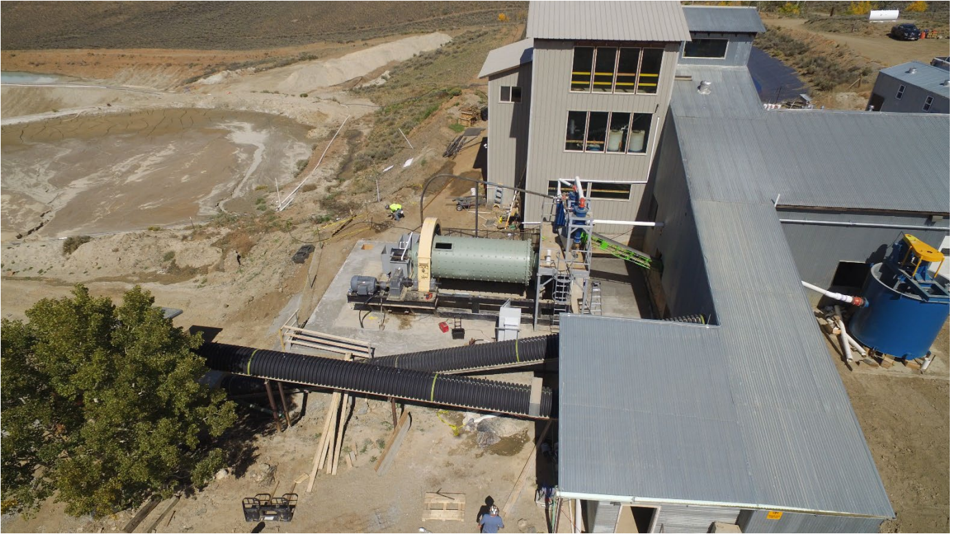
Figure 11: 250 tonne per day ball mill installed in place
