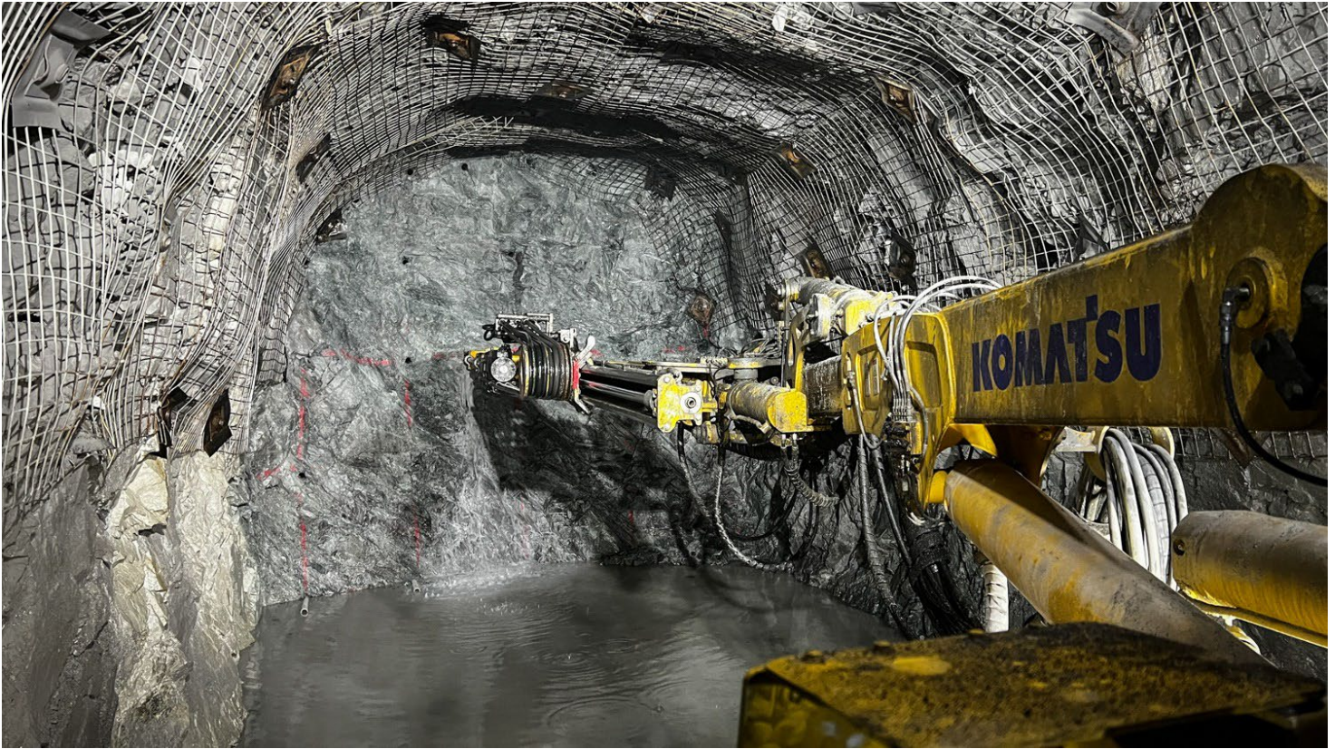
Figure 2 Komatsu Jumbo drill rig advancing the main decline
