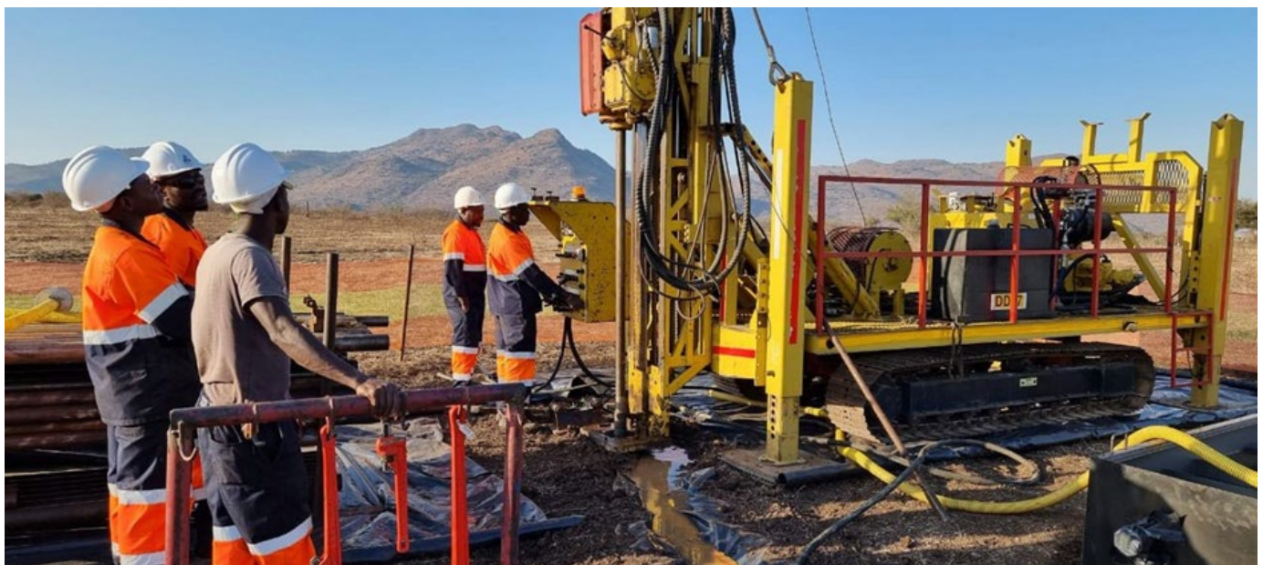
Figure 1: Atlas Copco drilling E019
