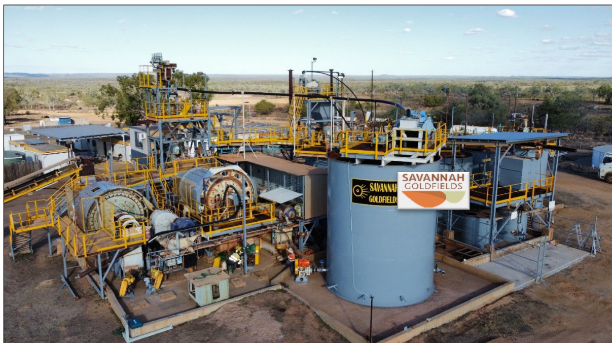
Georgetown Gold Processing Plant
