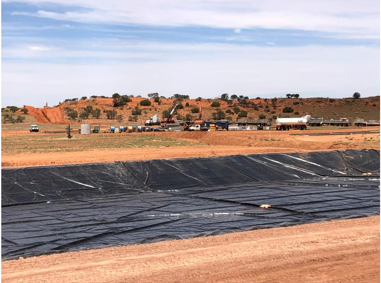
Installed pond liner with Vali-1 well site and laydown area
