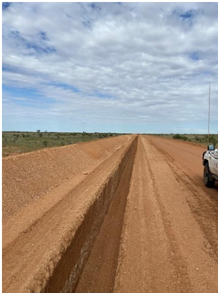
Completed trenching for installation of Fibrespar export line
