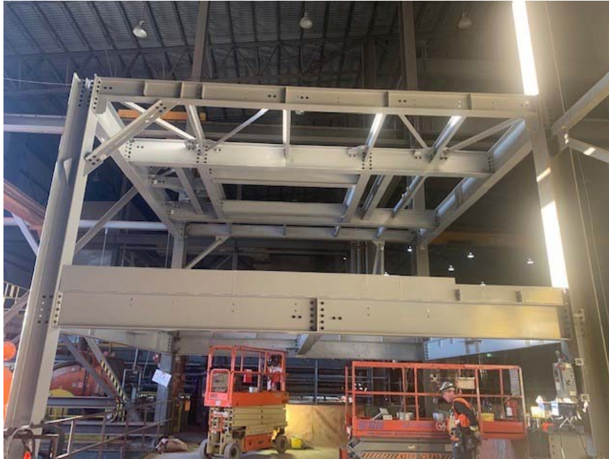
Figure 2: LIMS structure erection
