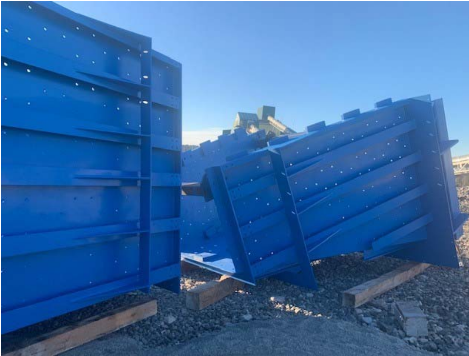
Figure 1: Dump Hopper components received at site
