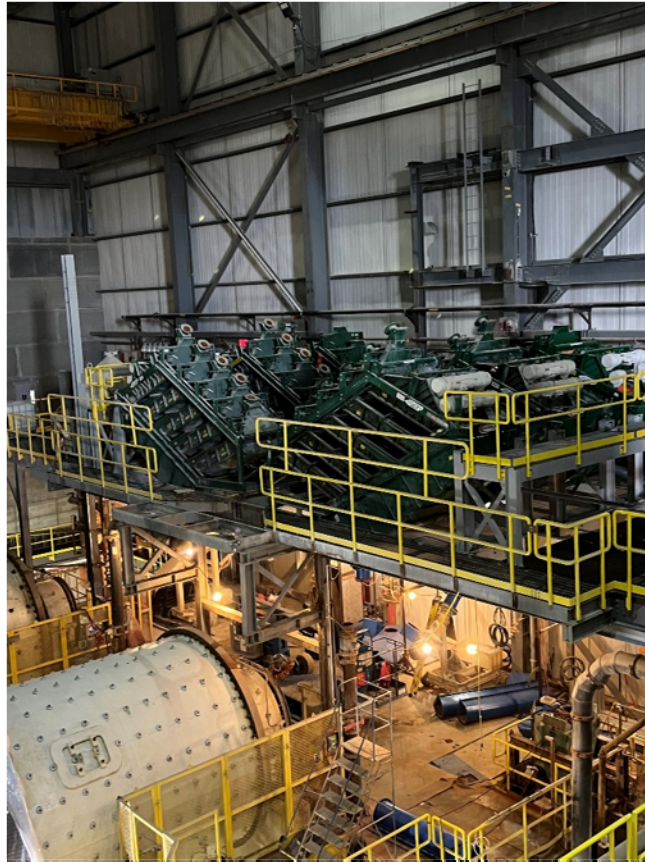
Figure 4: Derrick Screens installation
