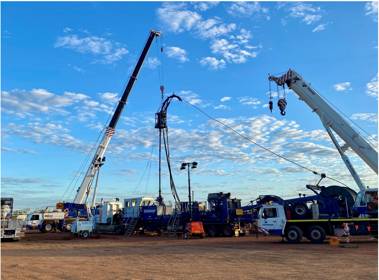
Rig up of the SLB frack spread at Carpentaria-3H
