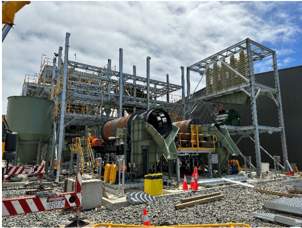
Figure 2 - Mechanical Installation of Ball Mills, Derrick Screens and Cleaner Spirals
