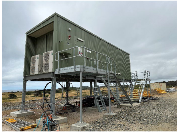
Figure 3 - Installation of Main Switch Room & Electrical Termination
