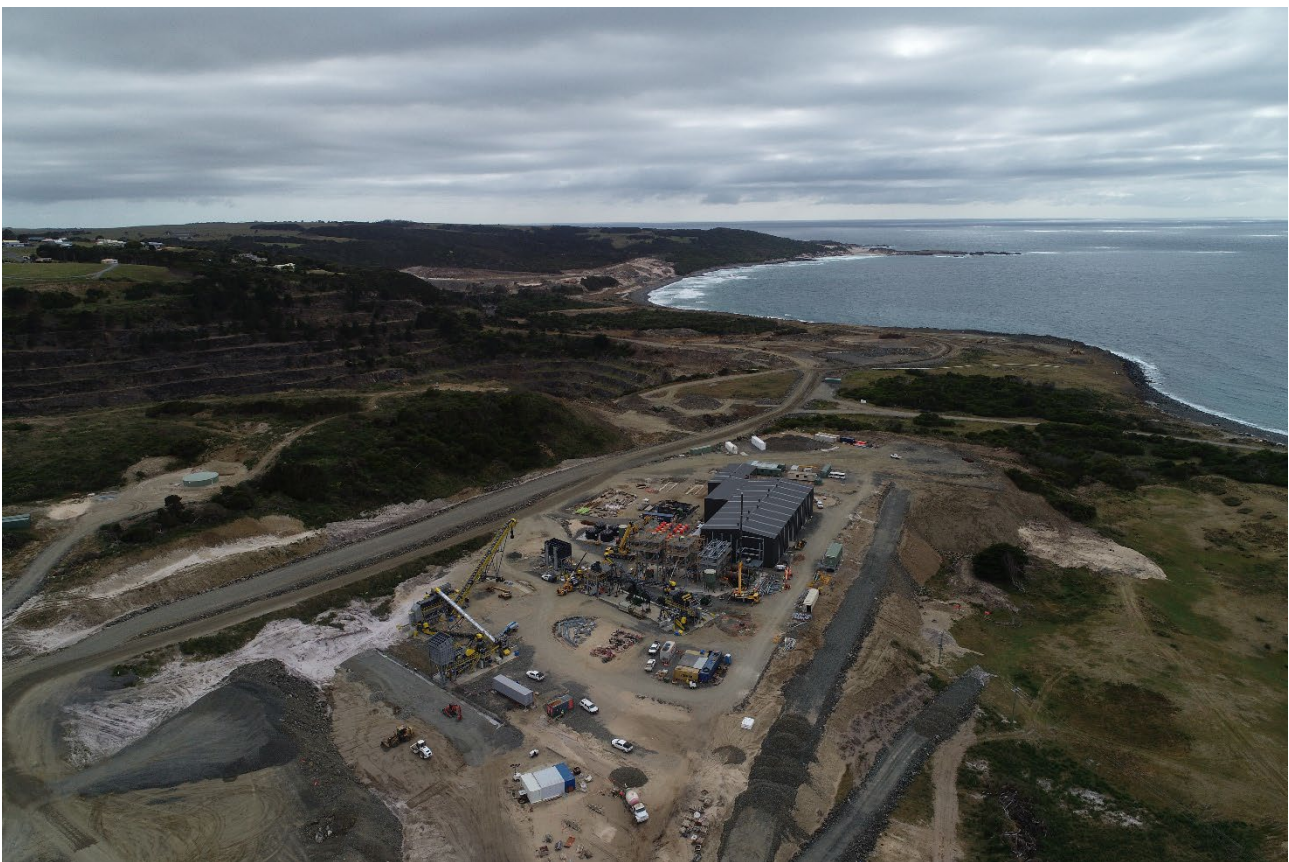
Figure 1- DTM Process Plant looking North-East
