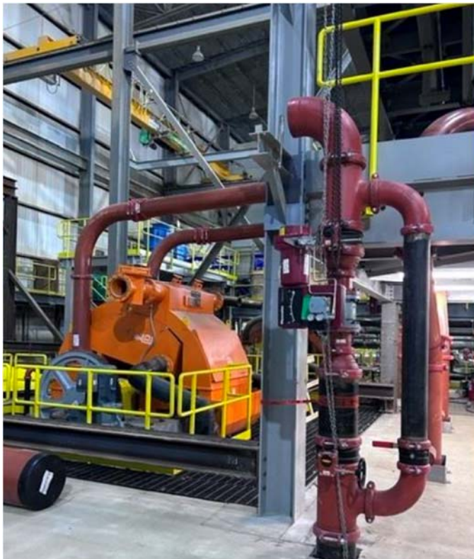
WHIMS piping installation
