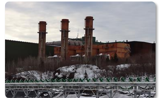
Pointe Noire Pelletizing Facility
