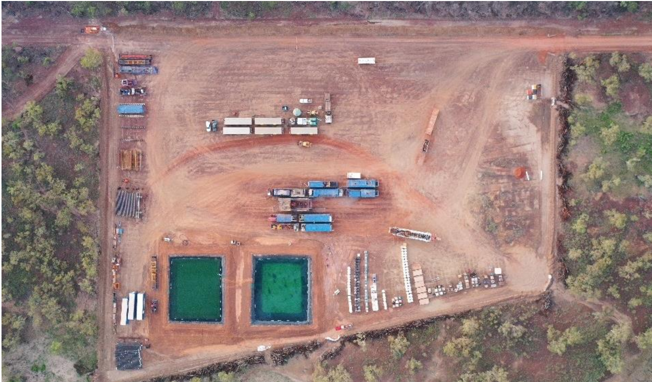
Carpentaria-4V site aerial view
