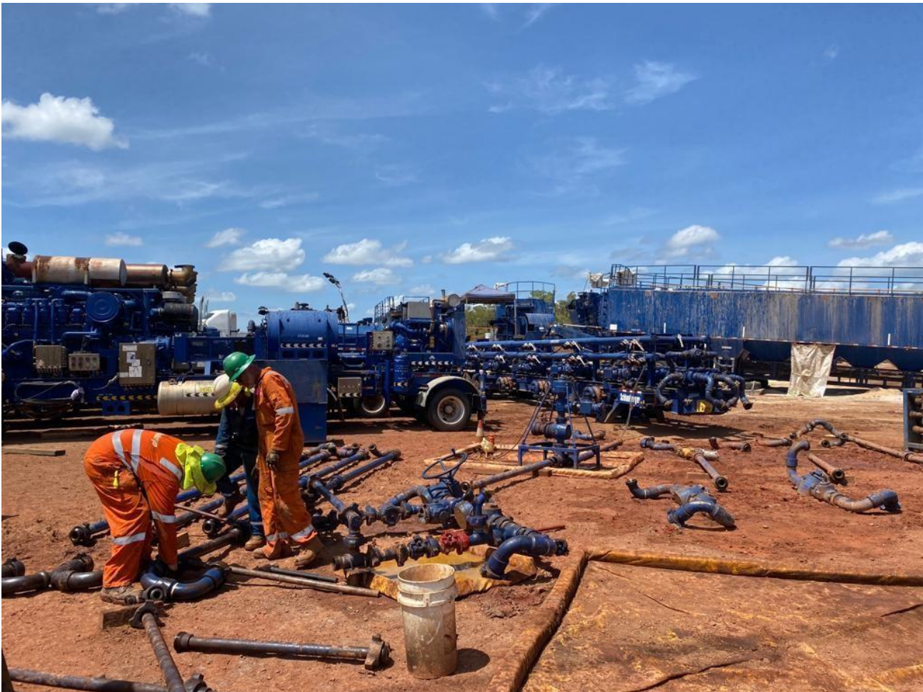
SLB crew rigging down high-pressure stimulation lines
