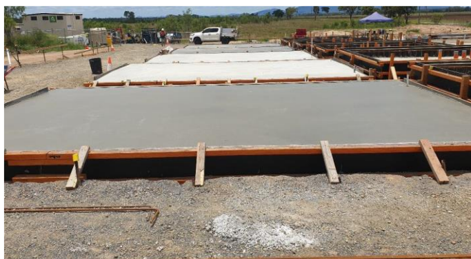
Figure 7: Megapack foundations
