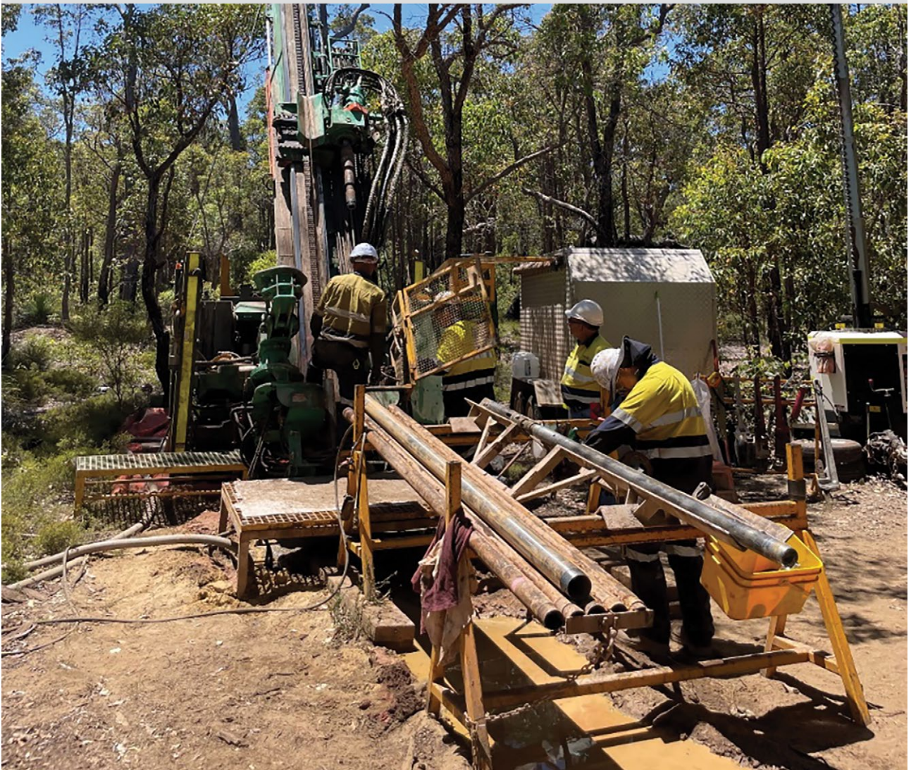
Figure 6: Diamond drilling underway at Greenbushes
