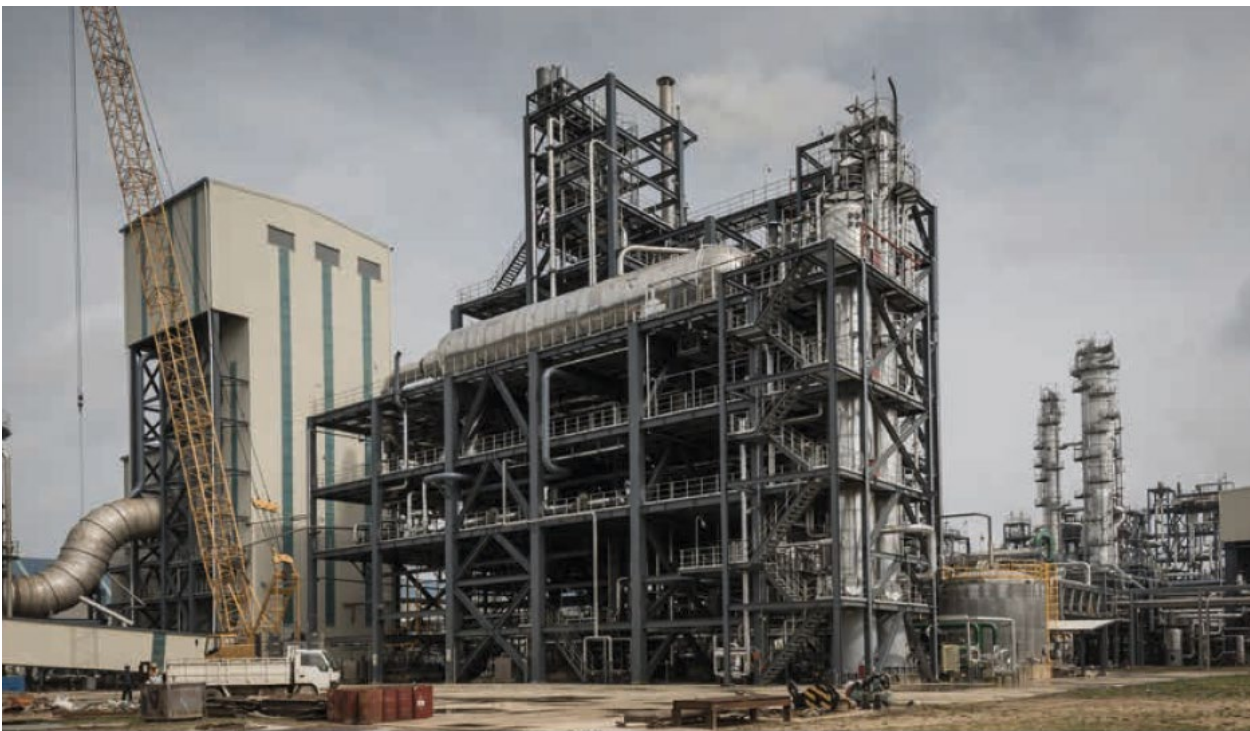
Photo 1: Typical Stamicarbon Urea Plant reactor
