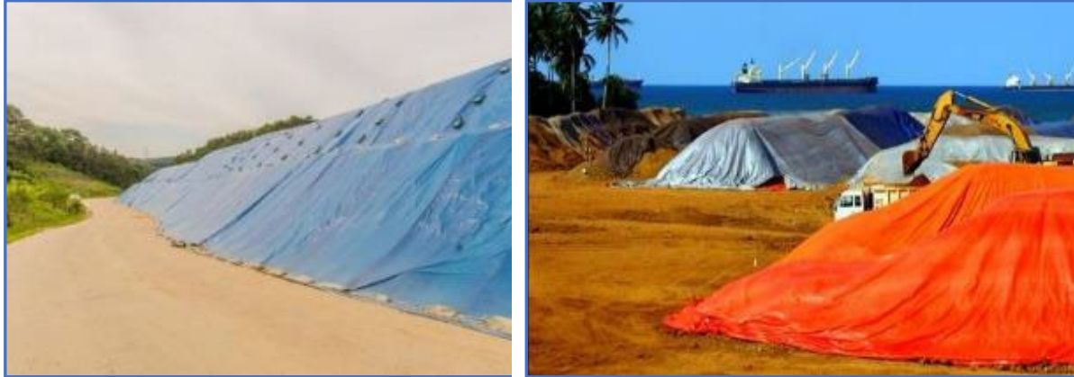
Figure 16 Typical Covered Stockpiles
