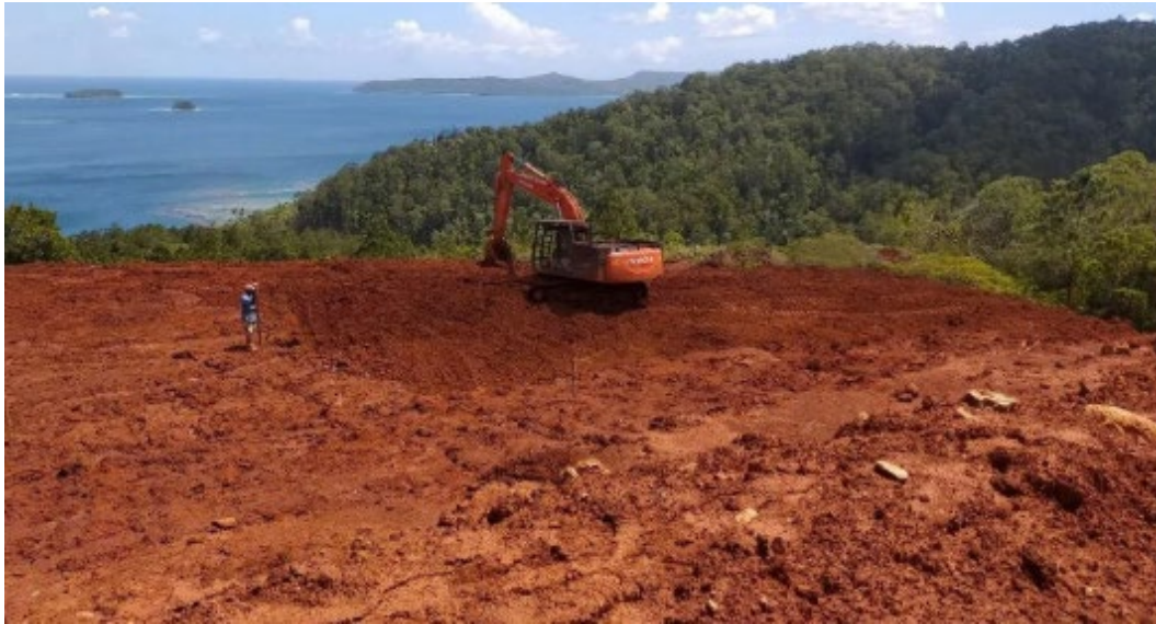
Figure 38 Pit Clearing and Access
