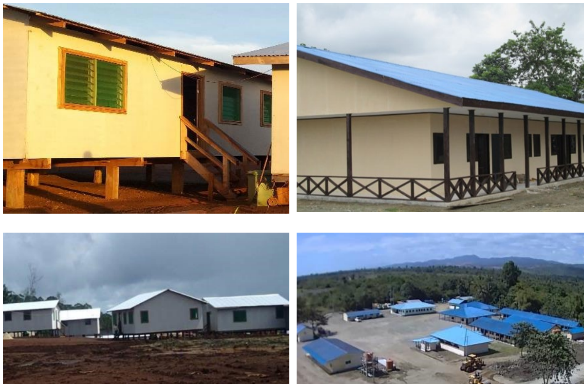
Figure 35 Local and Prefabricated Camp Buildings
