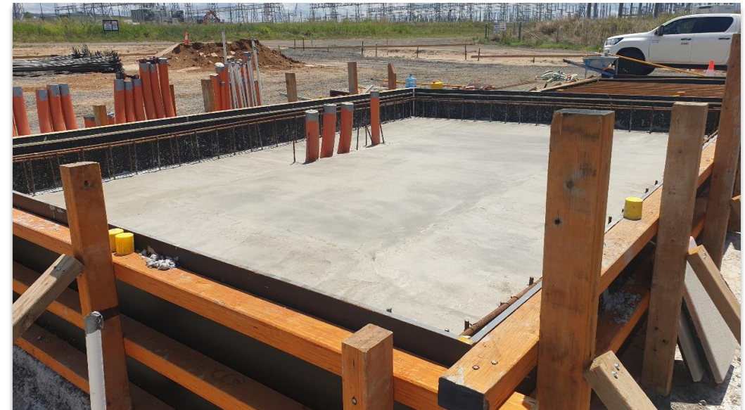
Figure: Step up transformer foundations
