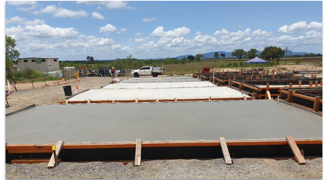
Figure: Megapack foundations
