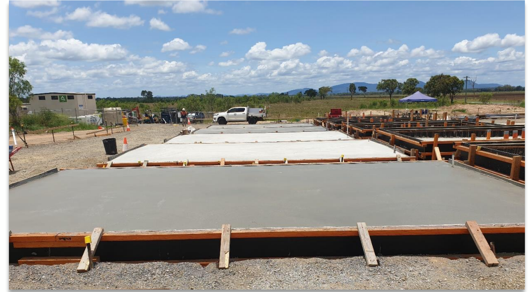
Figure: Megapack foundations
