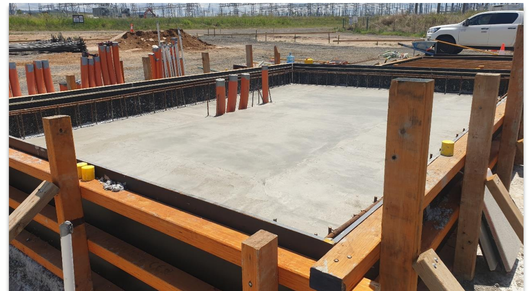
Figure: Step up transformer foundations
