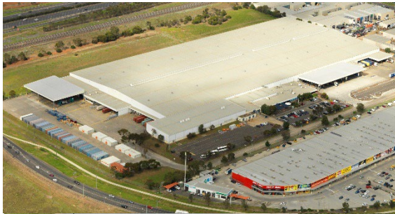
Woolworths Distribution Centre Hoppers Crossing, VIC
