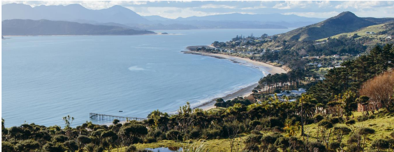
In December, the Hokianga Harbour community of Opononi was the last centre to be connected to fibre under our 11-year public-private partnership.
