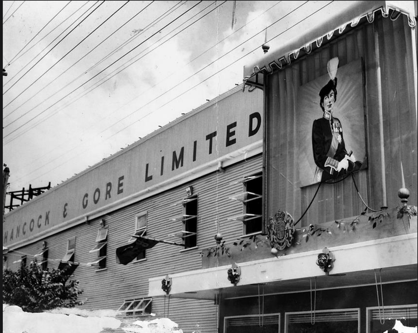
H&G Warehouse Ipswich March 1954
