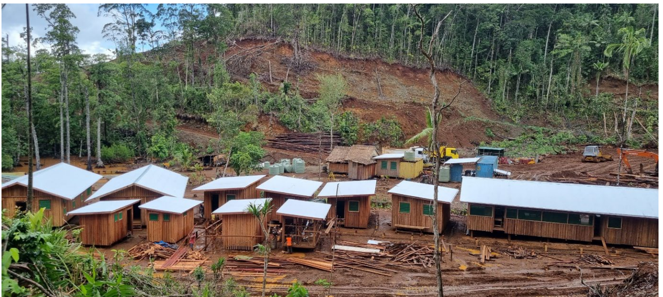
Photo 1: Construction of 50-man construction camp nearing completion
