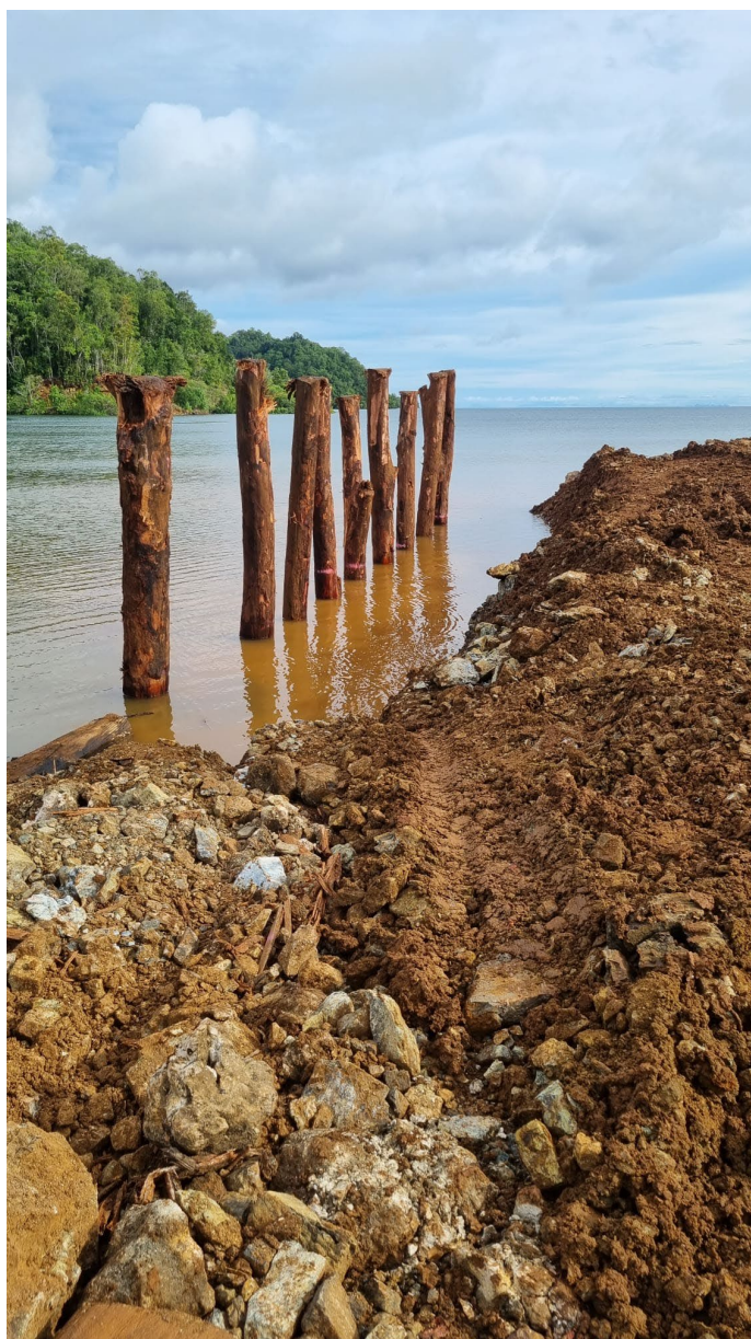
Photo 2: Construction of eastern face of DSO Loadout Wharf commenced
