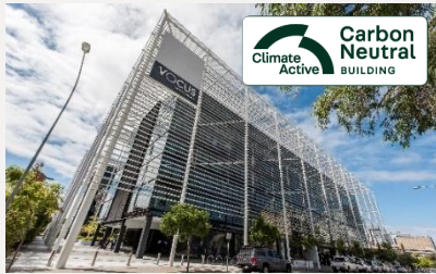
WorkZone West 202 Pier Street, Perth
