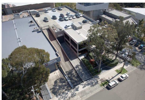
7 Sirius Road, Lane Cove NSW
