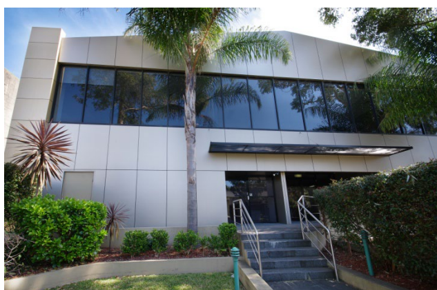
13 Sirius Road, Lane Cove NSW
