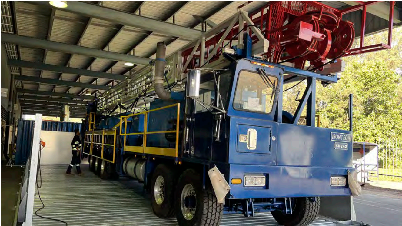
The new Rig and Well Services' wash bay in Withcott, Queensland.
