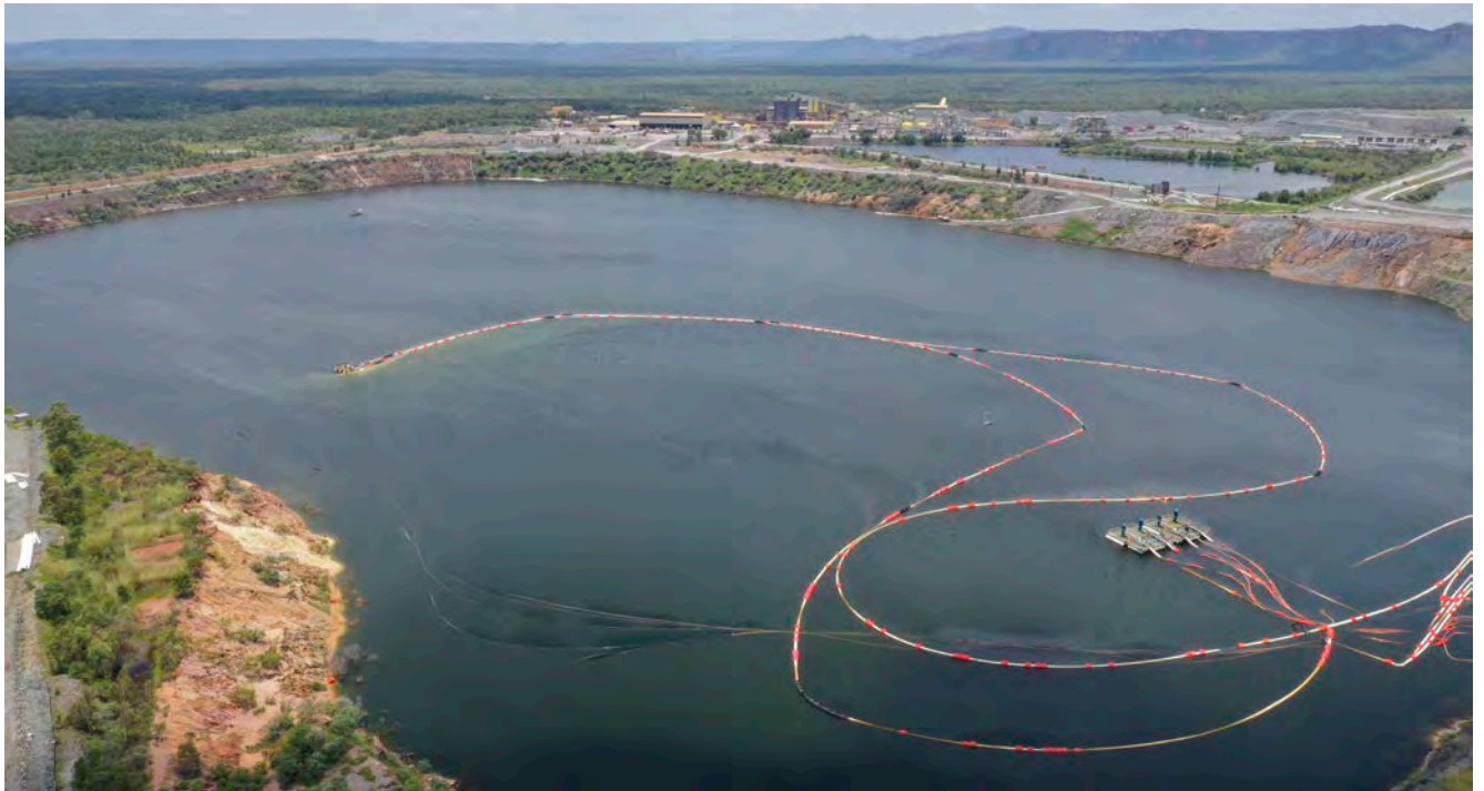
Prefabricated vertical drains (PFD) or 'wicks' being installed by Venita in Pit 3 at Ranger Mine.
