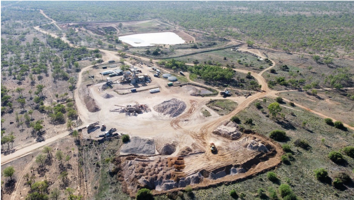
Georgetown Processing Plant and ROM stockpiles
