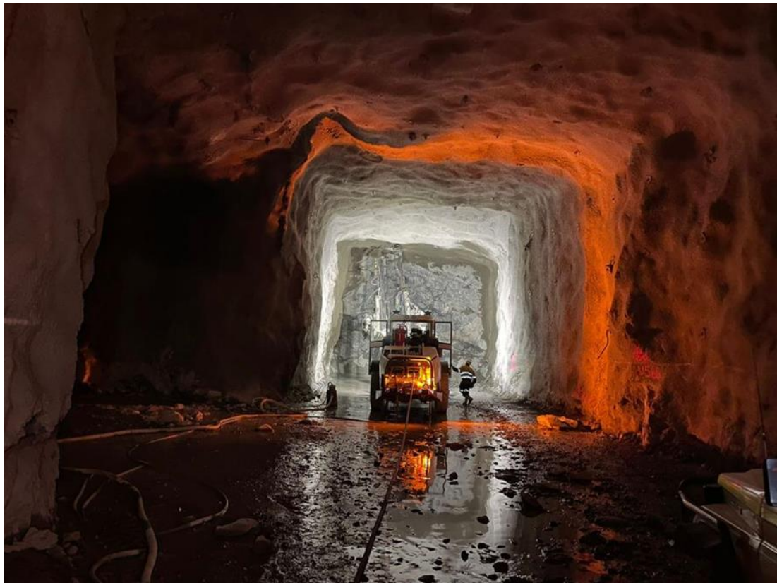
Figure 1: Powerhouse Cavern Excavation
