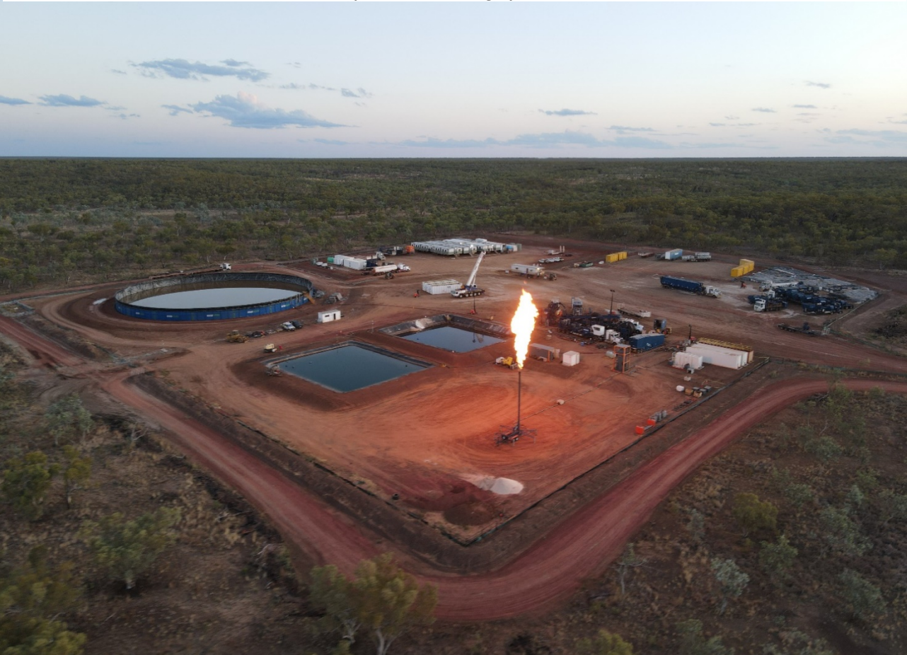
Carpentaria-2H Extended Production Test Flare
