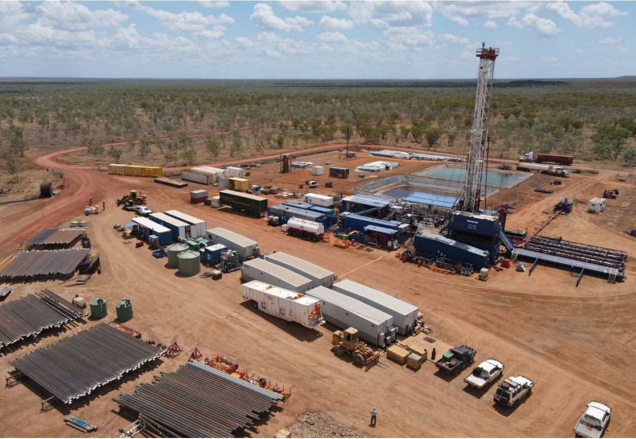
Carpentaria-3H Drilling Operations
