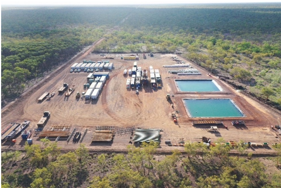
Carpentaria-4V Drilling Operations
