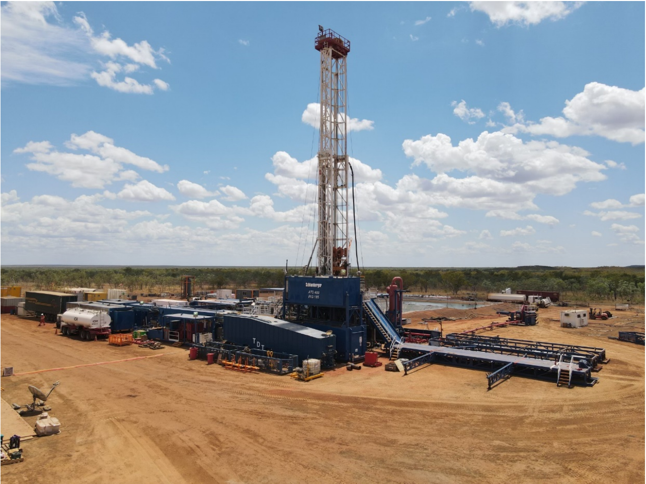
Carpentaria-3H Drilling Operations
