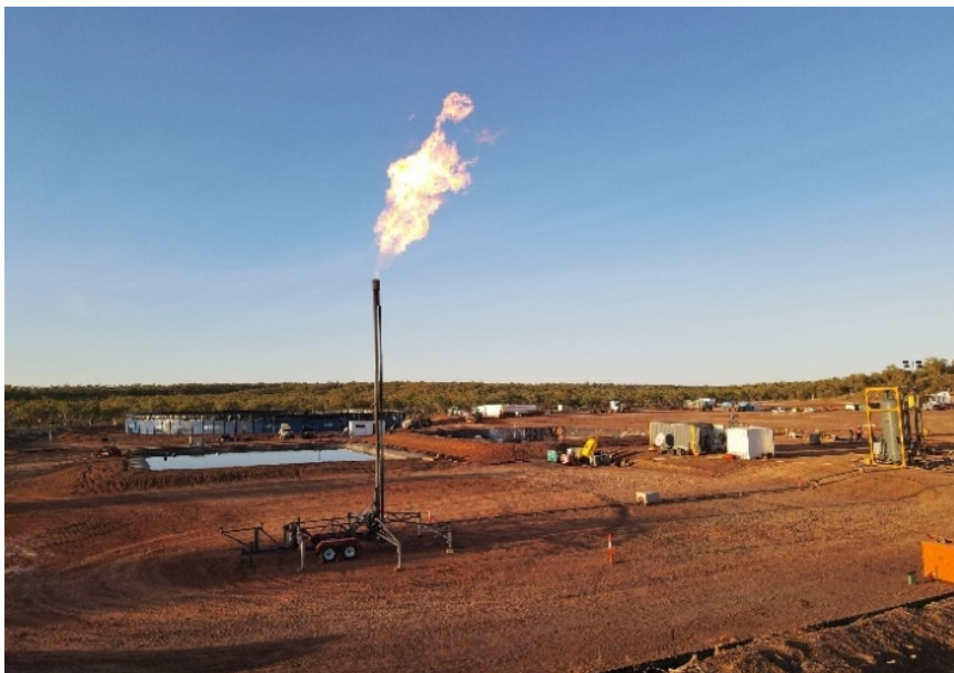
Carpentaria-2H Extended Production Test Flare
