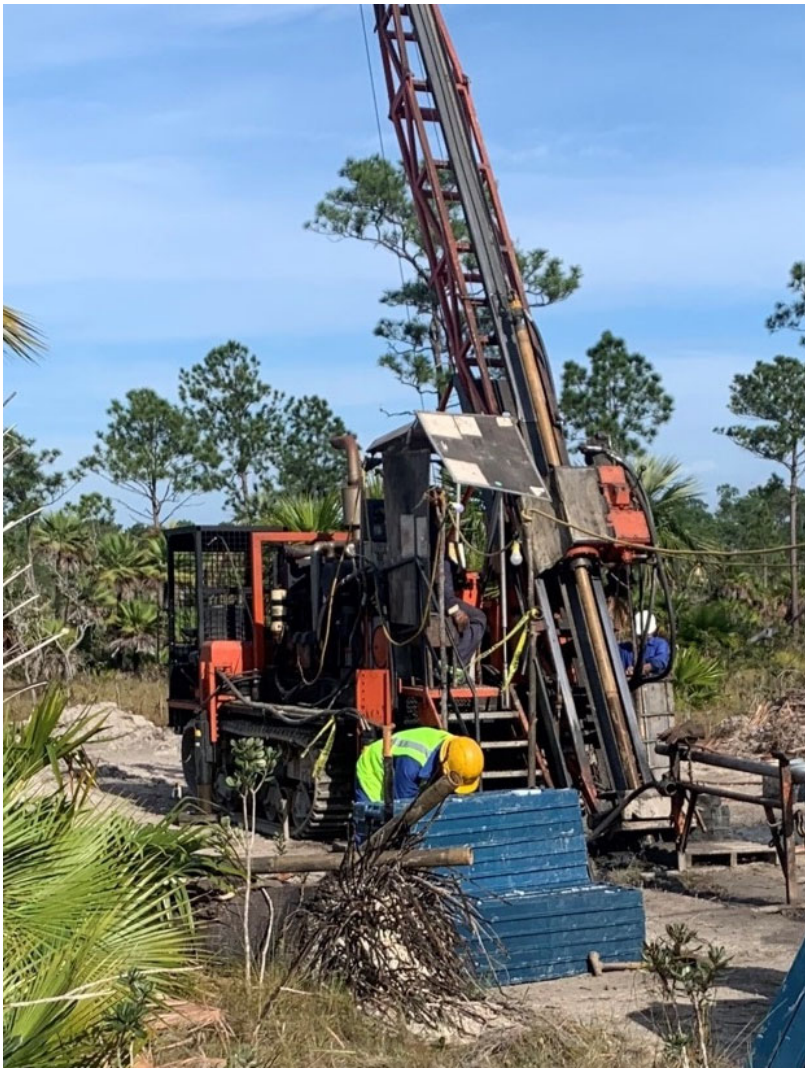
Drilling at La Demajagua
