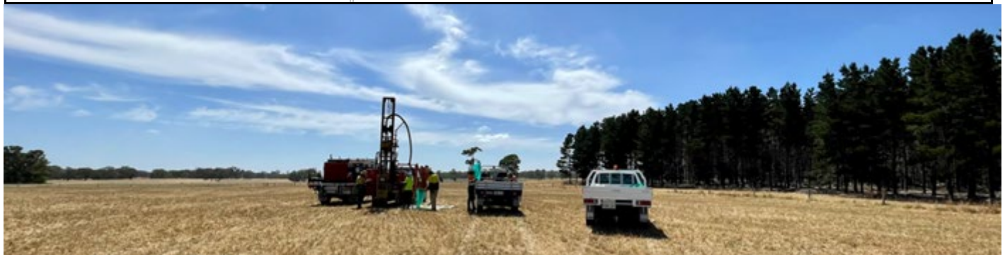
Drilling – Dovetail Region
