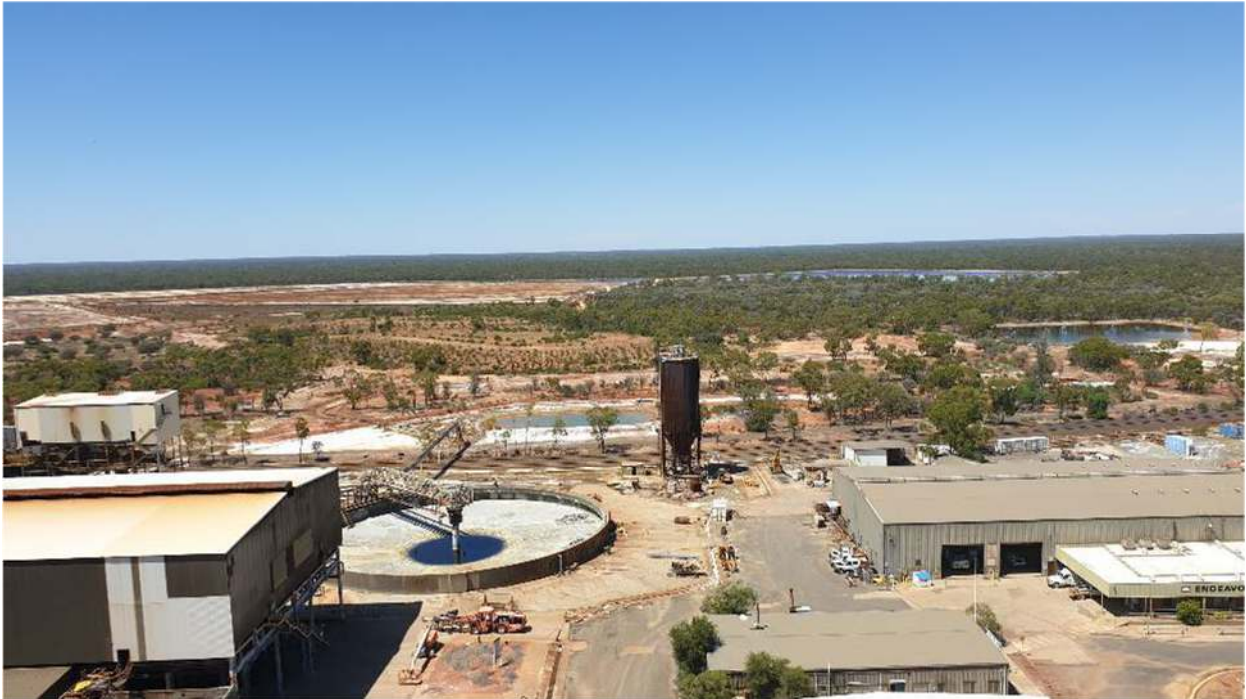
Photo 10 - Tails Thickener & Dam
