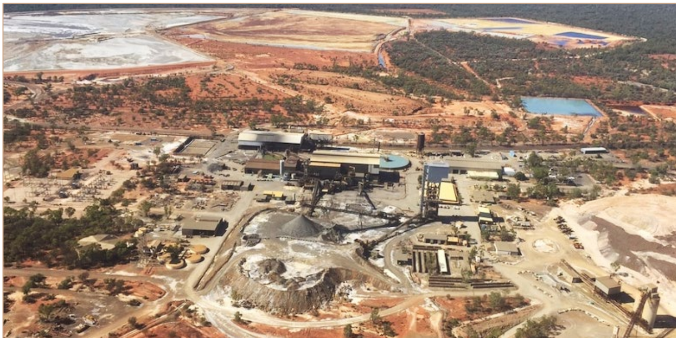
Figure 2: The Endeavor Mine – Surface Infrastructure (2019)
