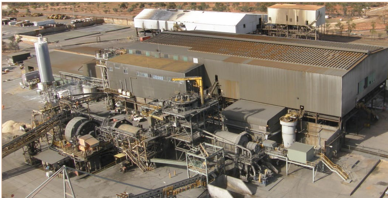
Figure 3: Endeavor Project: 1.2 MTPA Processing Plant (2019)
