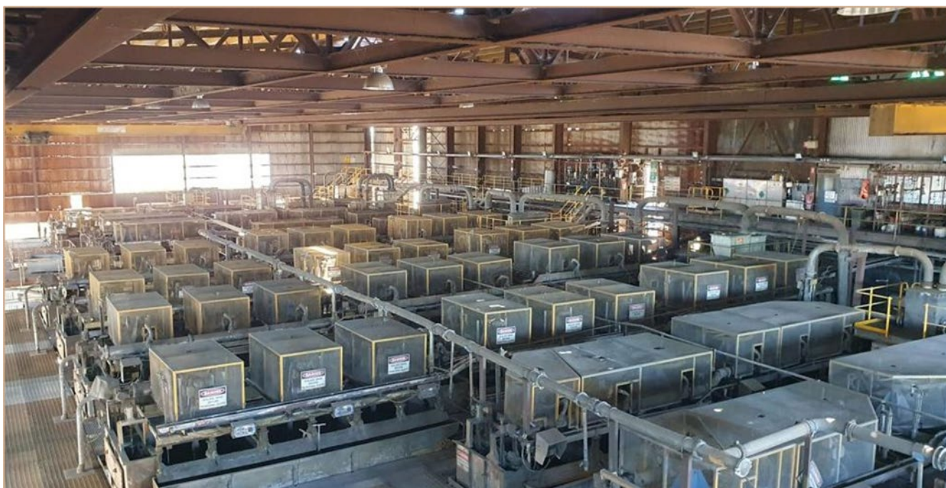
Figure 4: Endeavor – Lead / Zinc Flotation floor (February 2023)
