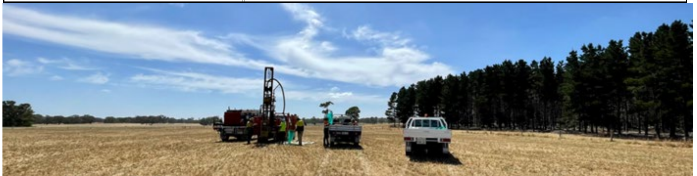
Drilling – Dovetail Region
