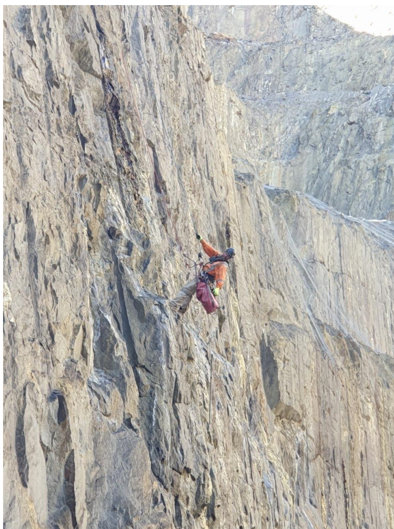
Figure 1 Installing mesh over pit walls
