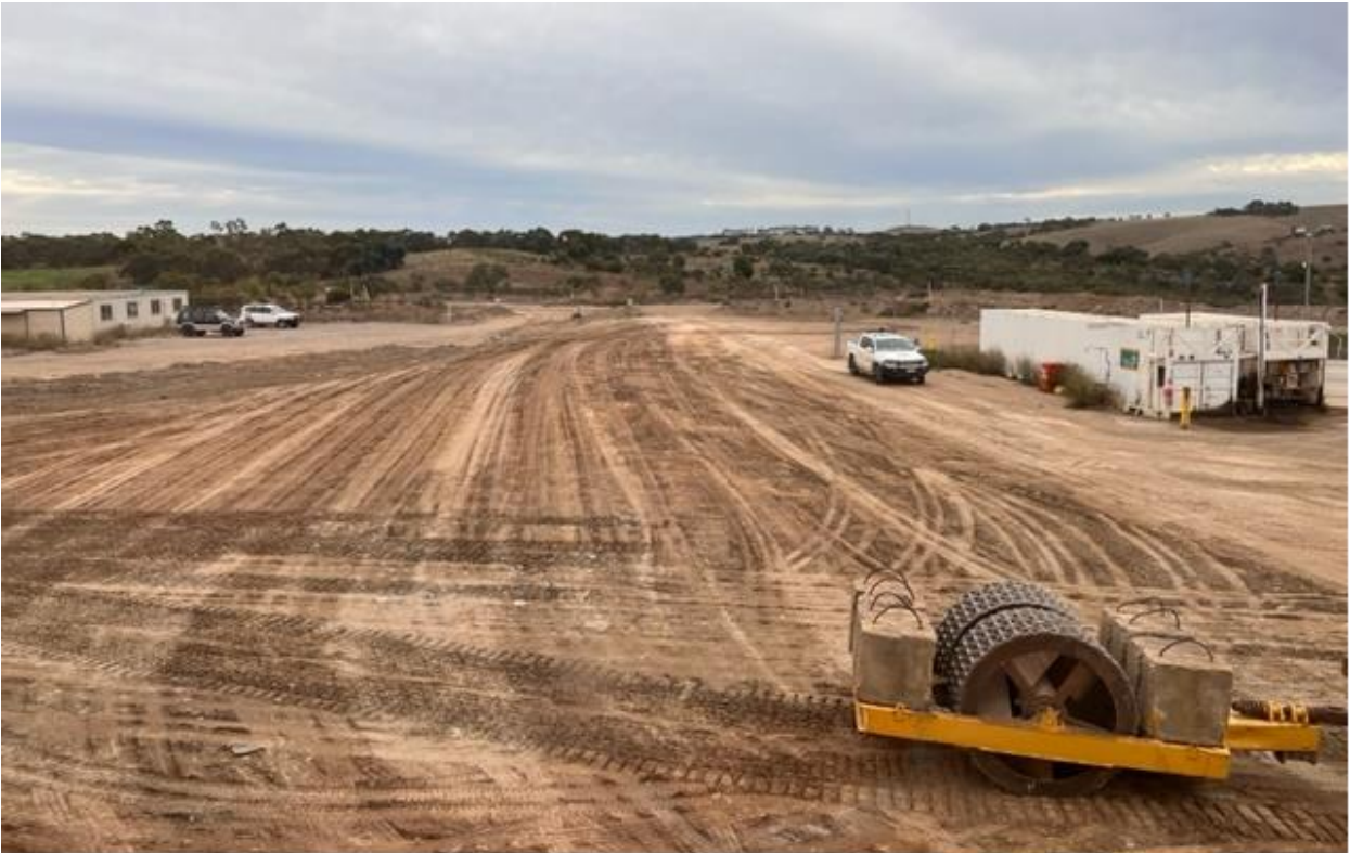
Figure 3 Preparing the change house area
