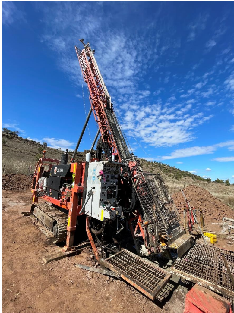
Figure 5 Exploration drilling underway in South Hub
