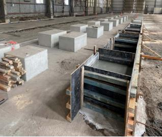
The vacuum pump slabs and pipe support footings have commenced with excavation and blinding completed and concrete slab pour planned in the coming weeks. The Spray Roaster has continued its progress with footing excavation and concrete works for slab and pedestals now complete. The civil works package remains on schedule to be completed by the end of April 2023.
