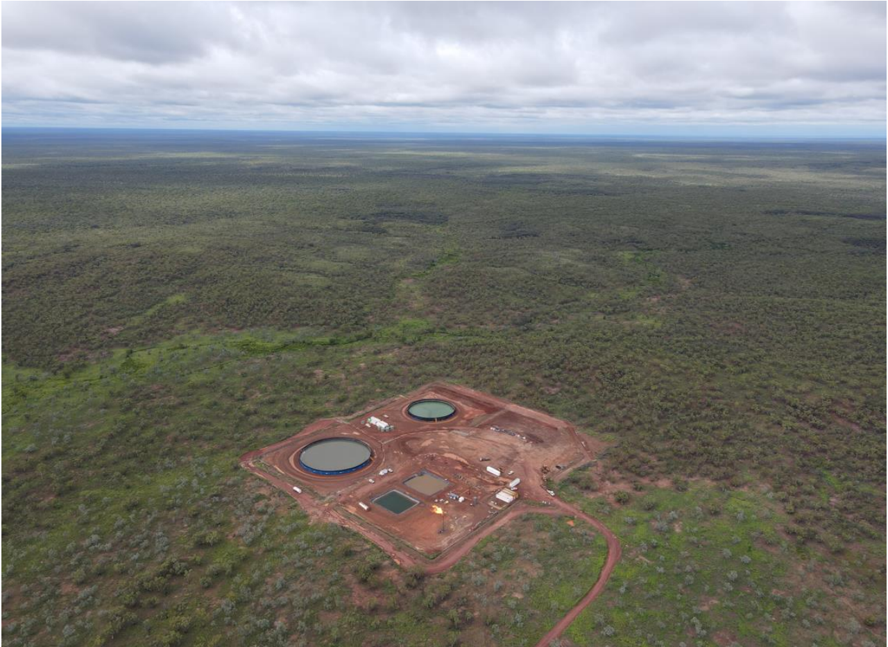
Carpentaria-3H wellpad from above
