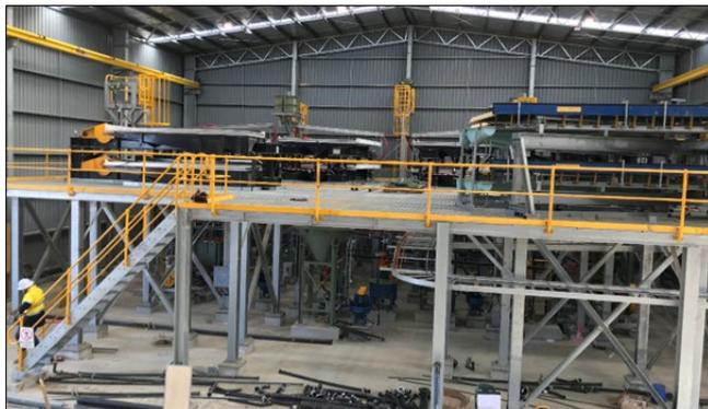
Figure 3 - View inside Process Building showing first floor gravity shaking table installation.
