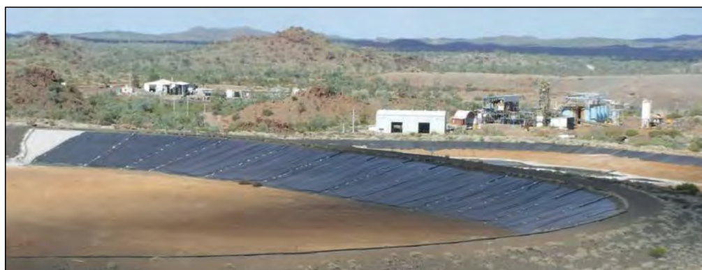
Figure 7-3. Overview of Great Australia process plant and infrastructure.
