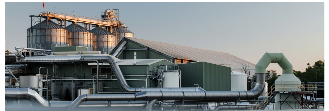
GrainCorp oilseed crush plant, Numurkah, Victoria
