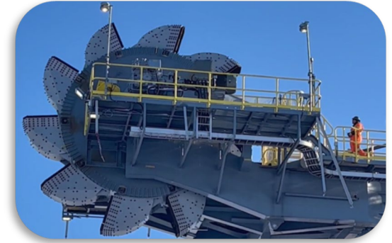
Progress on third-party infrastructure
