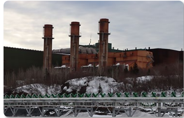
Pointe Noire Pelletizing Facility
