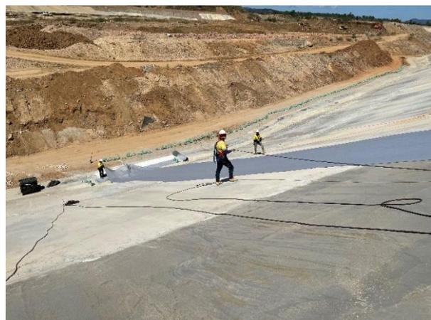
Figure 6: Installing the Geotextile Layer below the HDPE Liner
