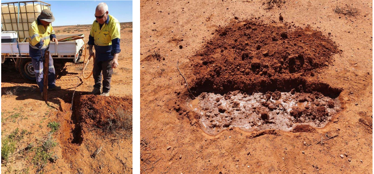
Digging and watering pit for electrode and prepared electrode in the ground
