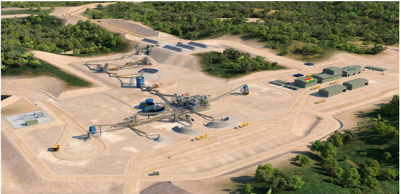
FIGURE 8 PROCESSING PLANT AND INFRASTRUCTURE VIEWED FROM THE WEST.
