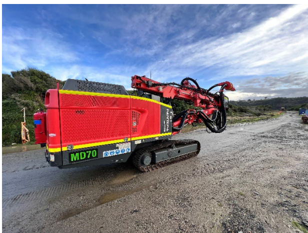
Figure 3 - Maxfield Drill & Blast Rig mobilised to site
