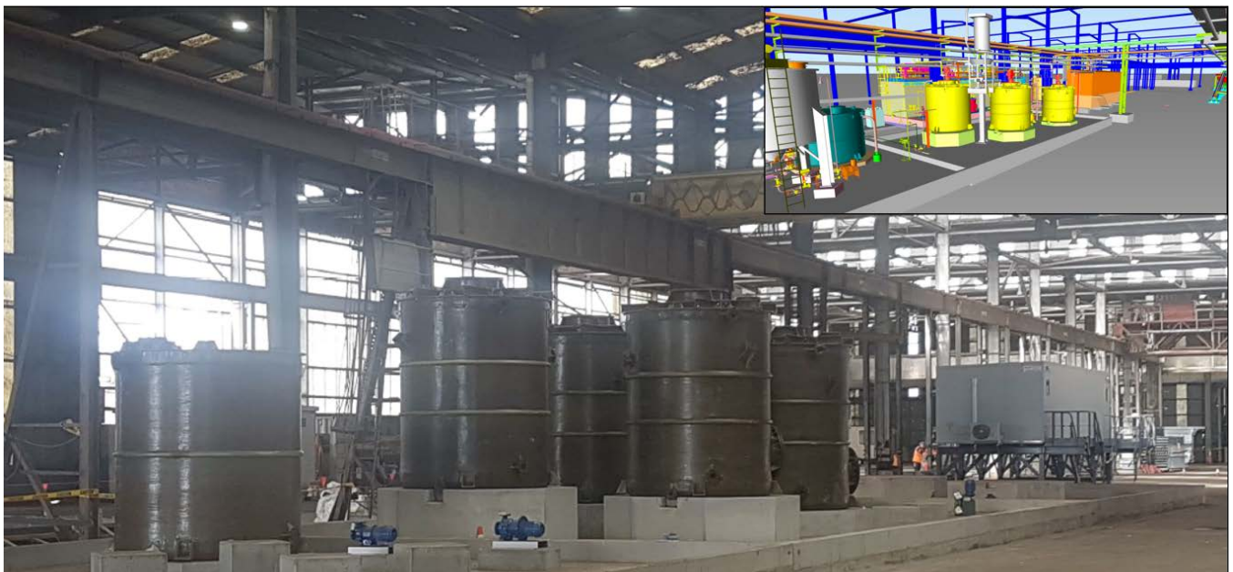
Figure: Impurity Removal FRP Tanks (top) and Reduction Area vacuum Pumps (bottom)
