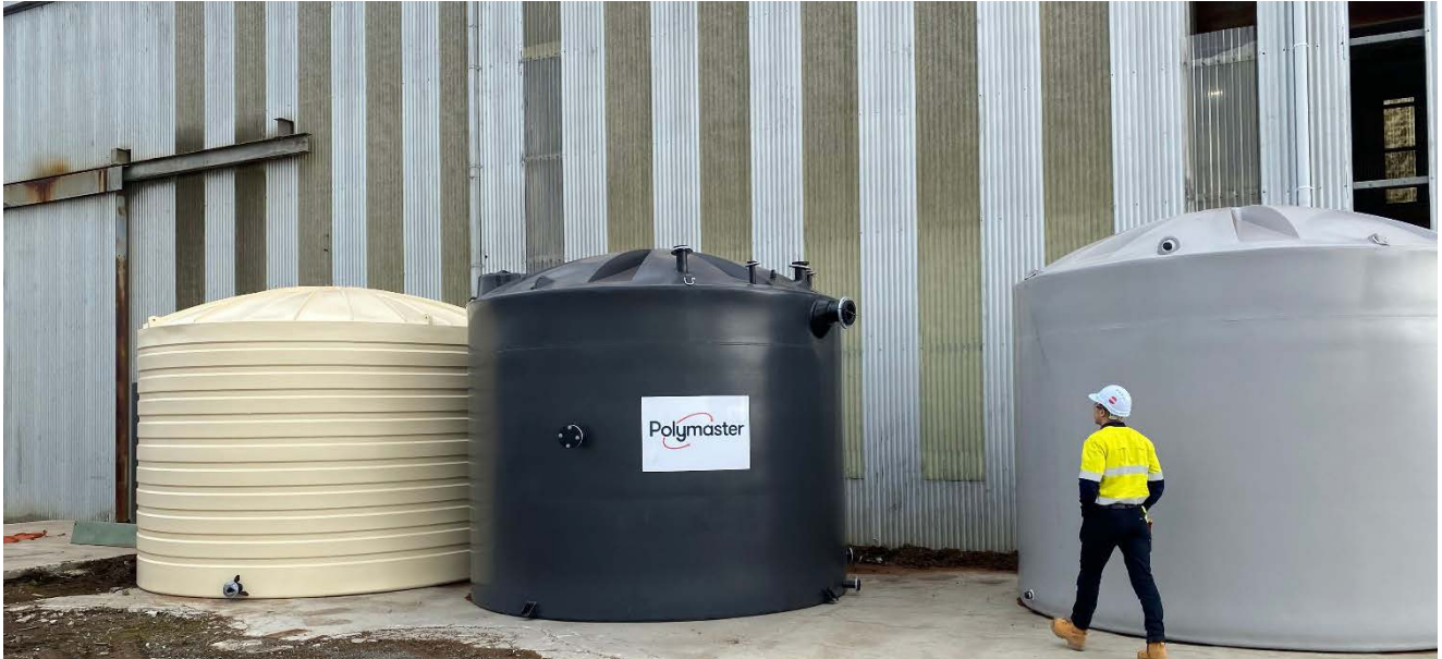
Figure: Raw Water (22.5kL), Process Water (27kL) & Brine Storage (18kL) Tanks On-Site
