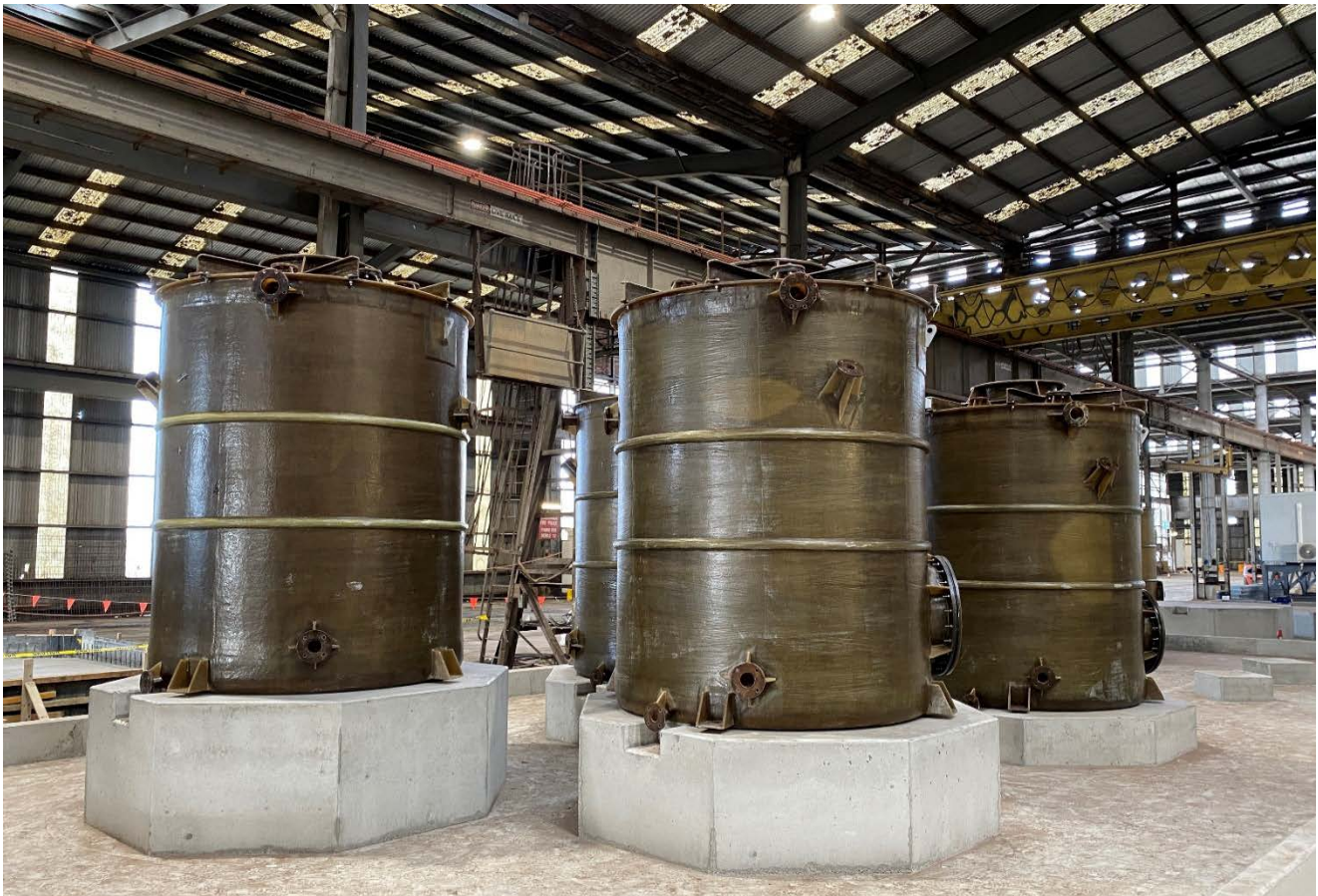
Figure: Installation of FRP Tanks on Plinths (top) and Delivery of Over-sized Tanks (bottom)
