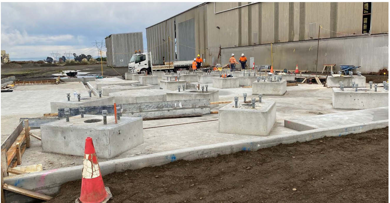
Figure: Spray Roaster Civil Works Package Completed
