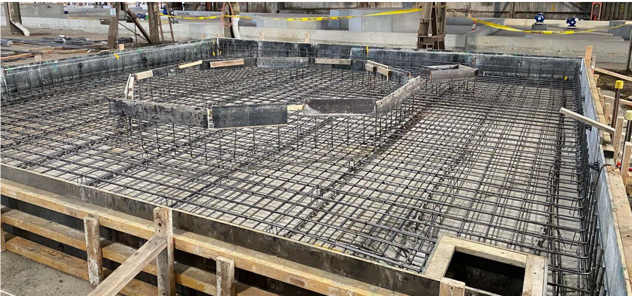
Figure: Magnesite Holding Tank Bund Reinforcement Complete
