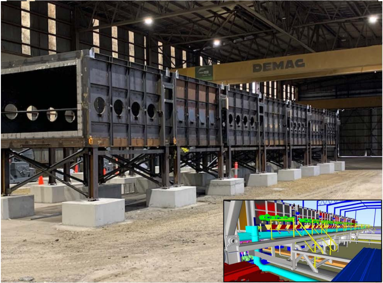
Figure: Installation of Reduction Furnace Modules (top) and Ash handling Conveyor System (bottom)
