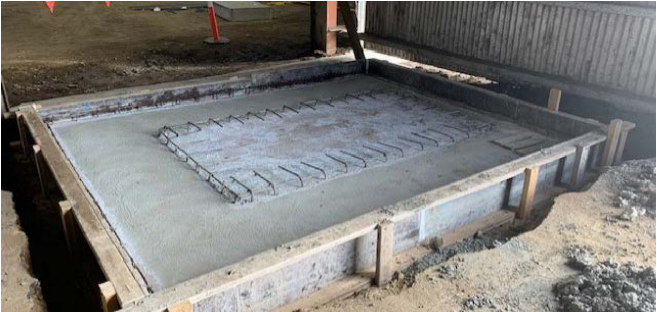
Figure: Scrubber Bund Prepared for Final Concrete Pour
