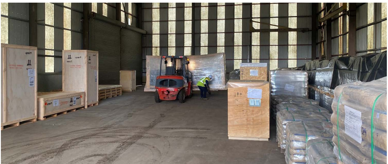
Figure: Process Control Software (PCS) Panel Delivery Stored Securely
