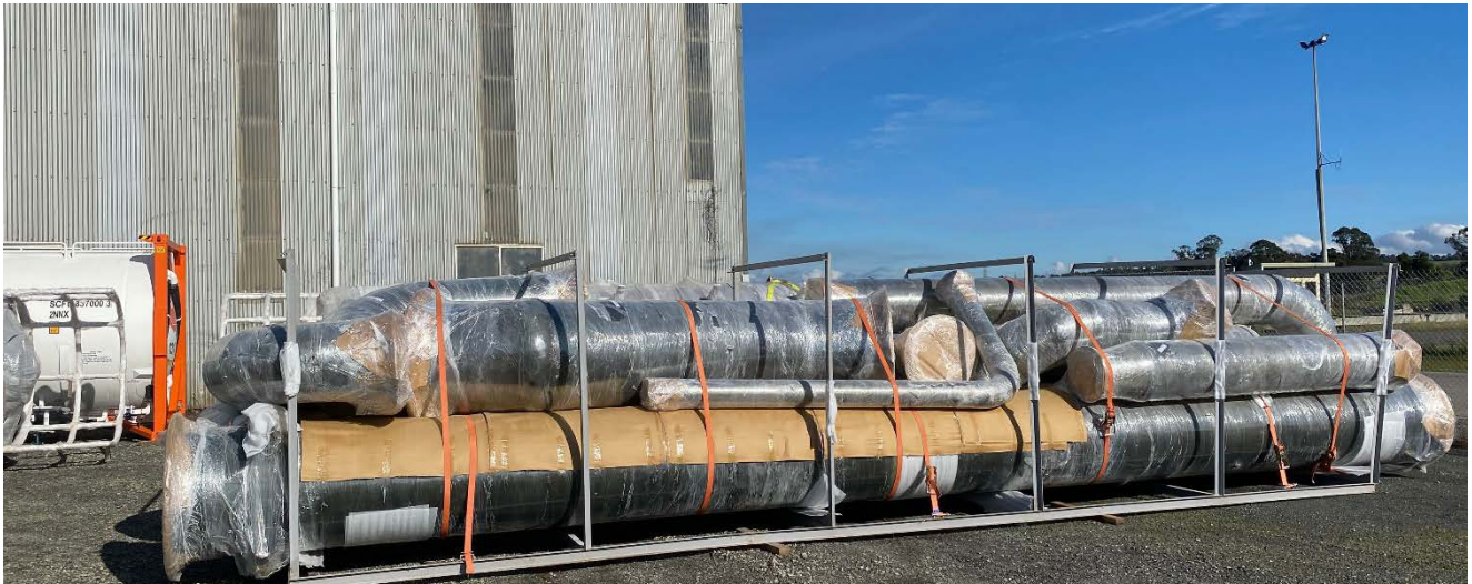
Figure: Spray Roaster Supplier Sub-Components Delivered On-Site
