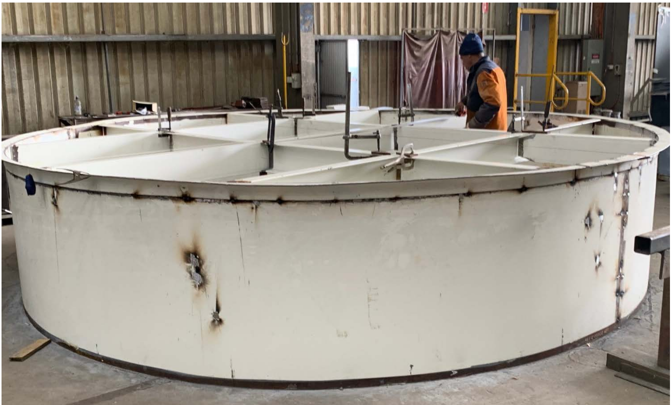
Figure: Workshop Fabrication of Spray Roaster Reactor Shell and Oxide Bin
