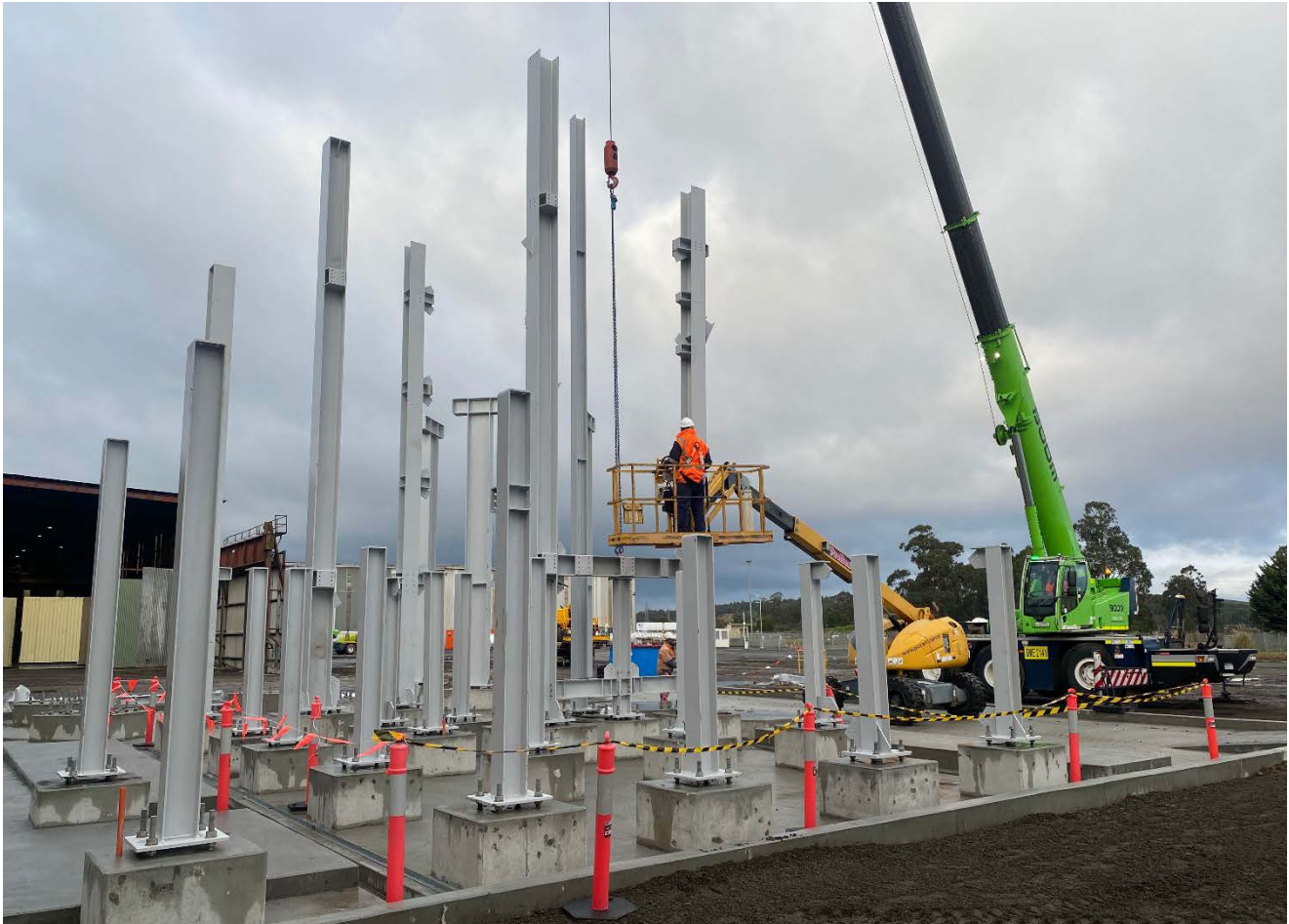
Figure: Spray Roaster Structural Steel Erection (top) and Level 1 Erection Complete (bottom)
