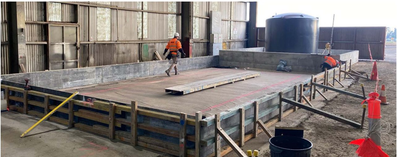
Figure: Process & Raw Water Bund Formwork for Bund Walls
