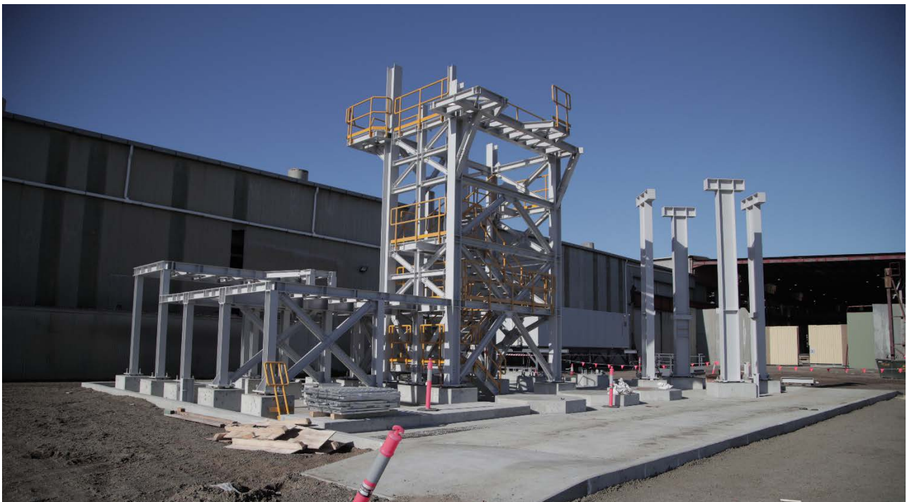
Figure: Spray Roaster Structural Steel Erection (top) and Level 1 Erection Complete (bottom)
