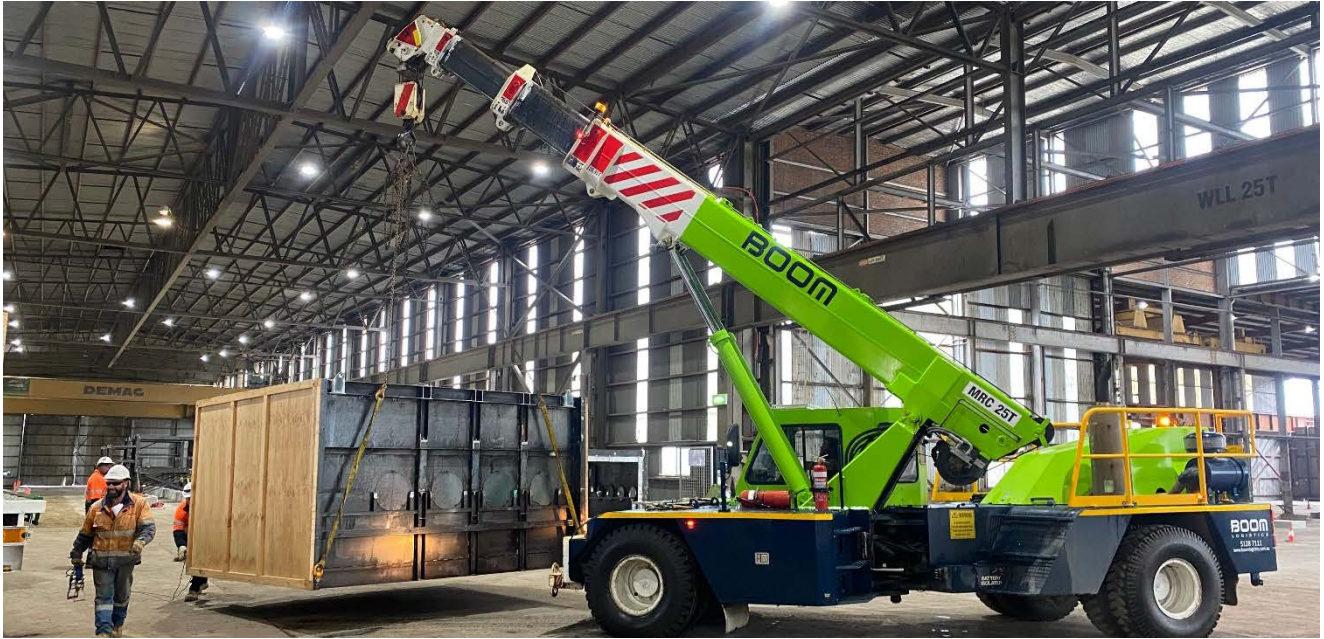
Figure: Reduction Furnace Module Delivery Unloading
