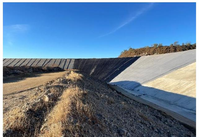
Figure 5: Wises Dam Liner Installation
