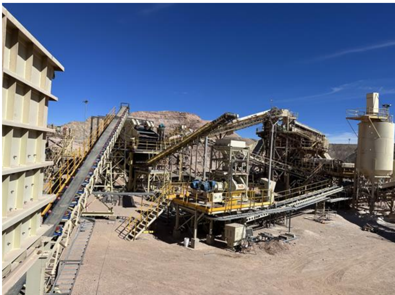
New Crusher facility at the Guanaco-Amancaya Mine Complex (Chile)
