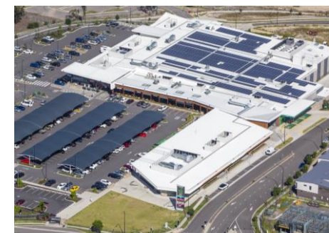
CAMERON PARK PLAZA, CAMERON PARK NSW
