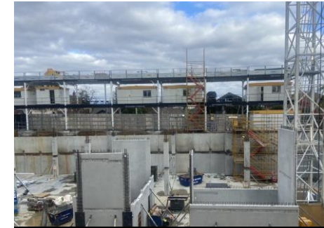
PROGRESS PHOTO - ADENEY PRIVATE HOSPITAL, KEW VIC
