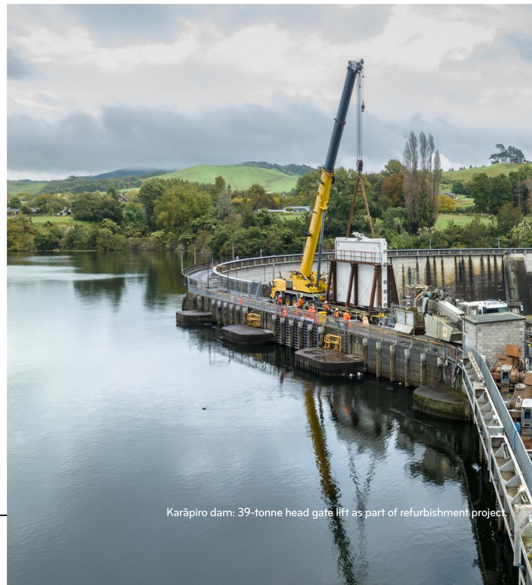
Karāpiro dam: 39-tonne head gate lift as part of refurbishment project.
