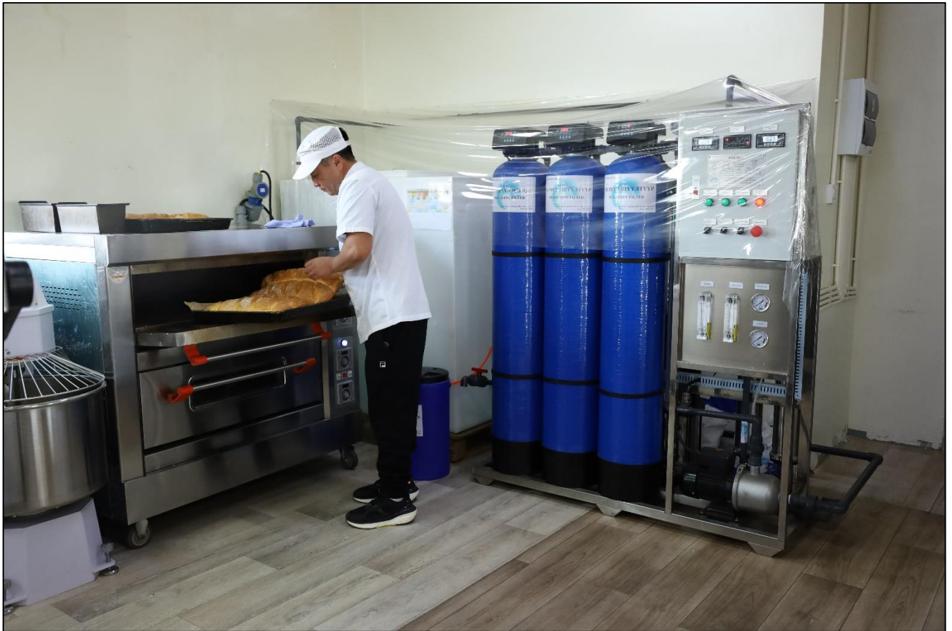
Figure 5: New Kharmagtai Water Filtration Systems
