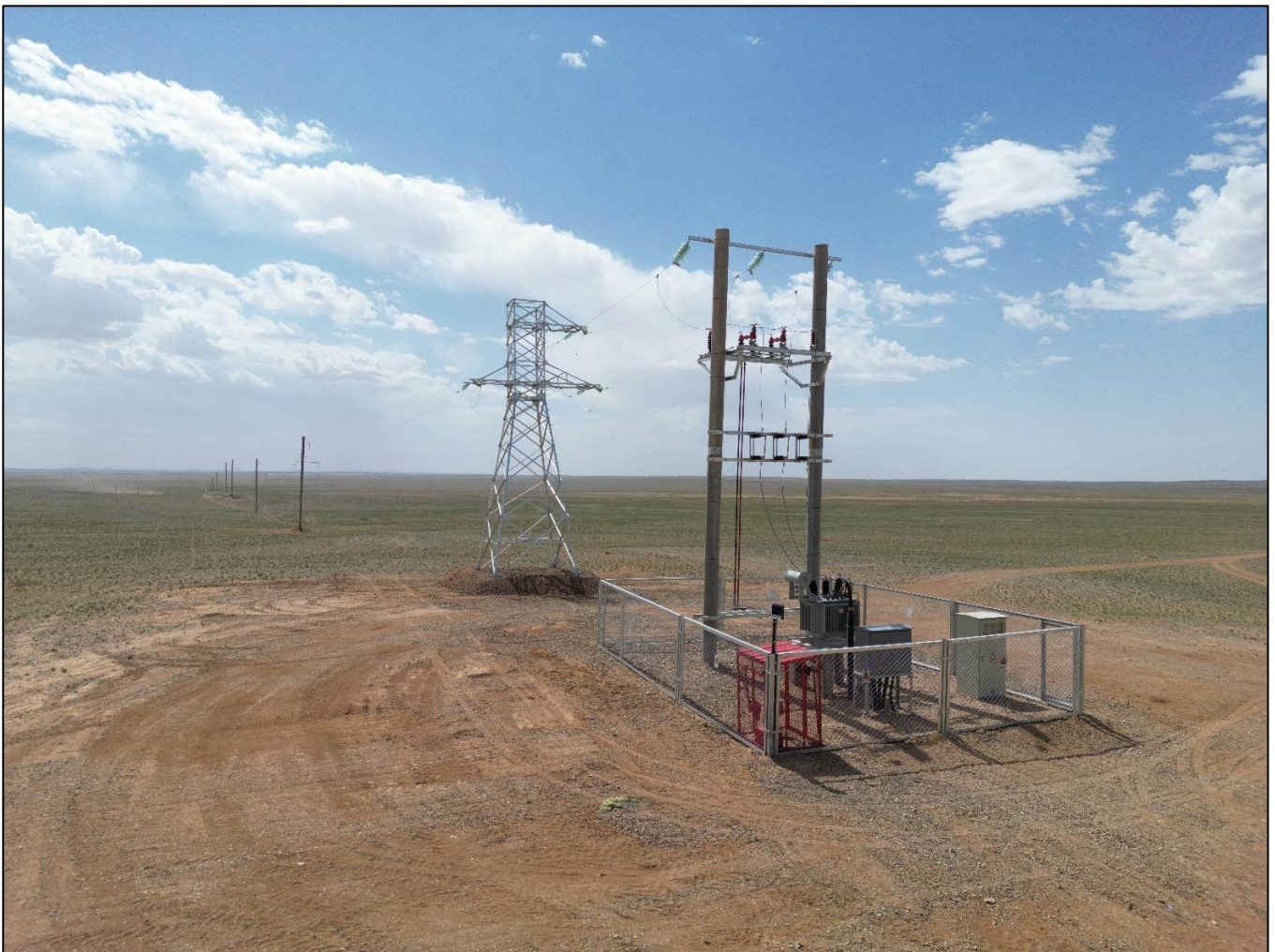
Figure 1: 35kV connection to Mongolian SEDN grid.
