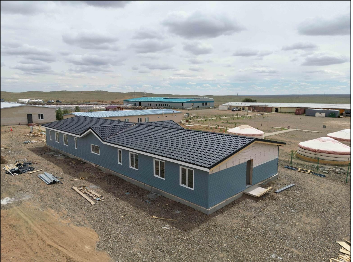
Figure 3: New Accommodation Block under construction.
