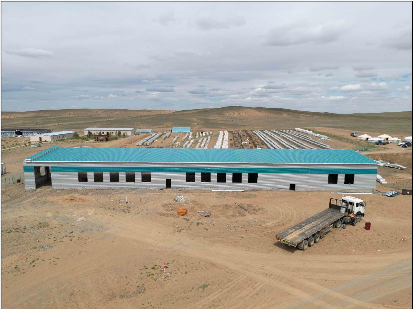
Figure 2: New Core Processing Facility under construction
