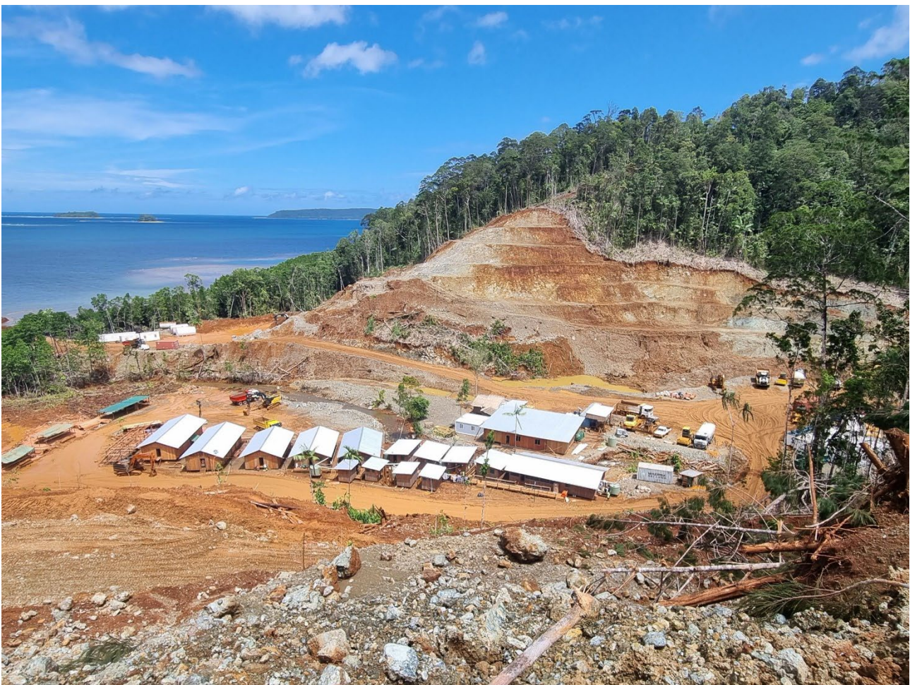
Photo 4. Camp and project offices
