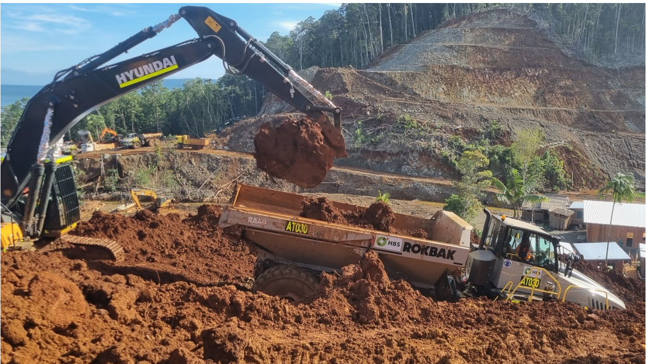
Photo 2. HBS RokBak articulated truck being loaded, working on haul road
